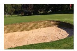
Bunker aesthetics can be dramatically changed by the way our turf is stacked. Double stacking, which results in a typical revett thickness of 40mm (1.6 inches) is the default setting for most of our projects and works well on both inland parkland projects and seaside links. However there are times when a single stack is needed to create a beautiful smooth face (such as Killara GC) or a triple stack, very popular in Scotland, where a bold layered aesthetic is desirable.
